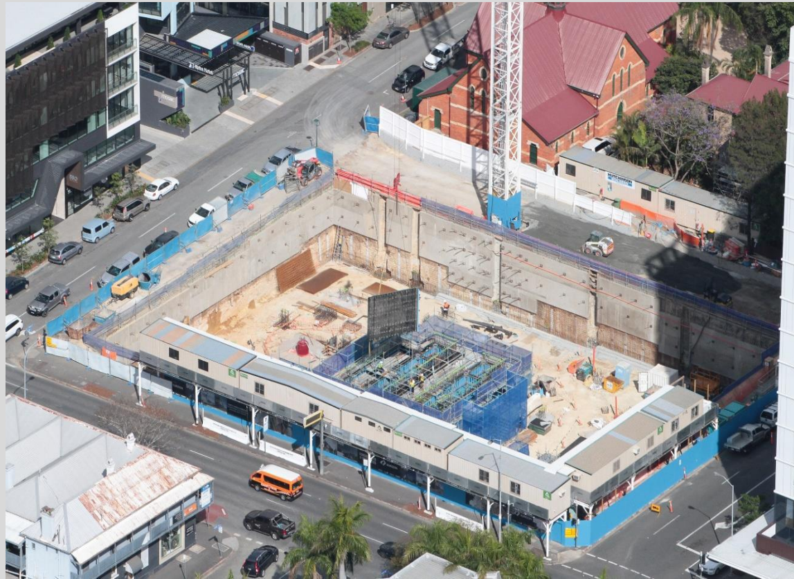
Construction progress as at December 2016
