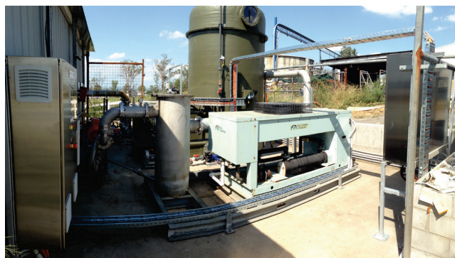
AJ Bush engine pre installation and gas conditioning equipment including biological scrubber.
