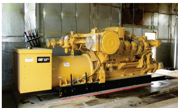
AJ Bush engine pre installation and gas conditioning equipment including biological scrubber.
