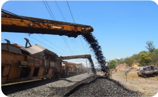
Ballast Undercutting Machine in Operation
