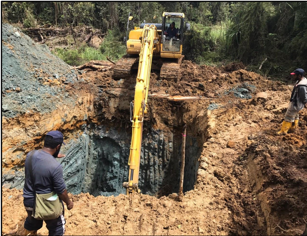
Photo 1: Excavator digging bulk sample Pit 200 at Crown Ridge
