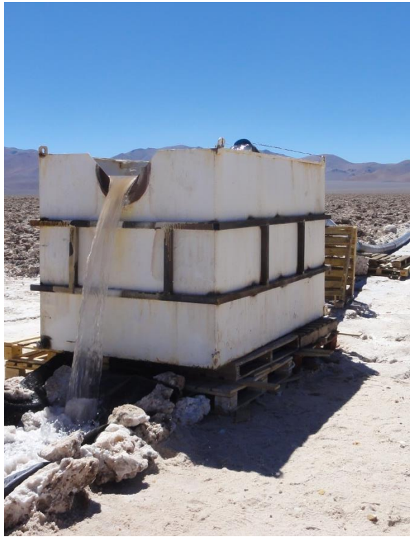
Figure 4: P4 pump test discharge point
