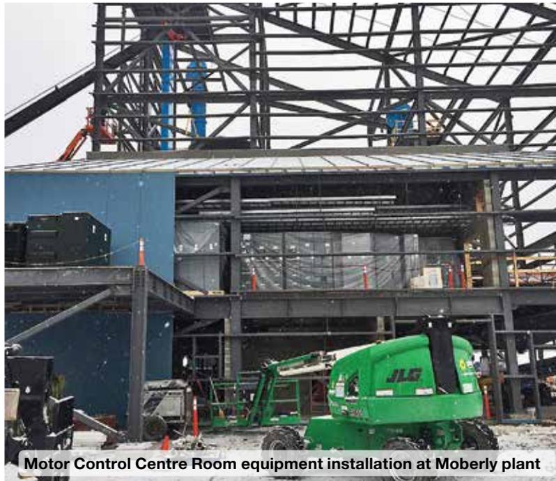
Motor Control Centre Room equipment installation at Moberly plant
