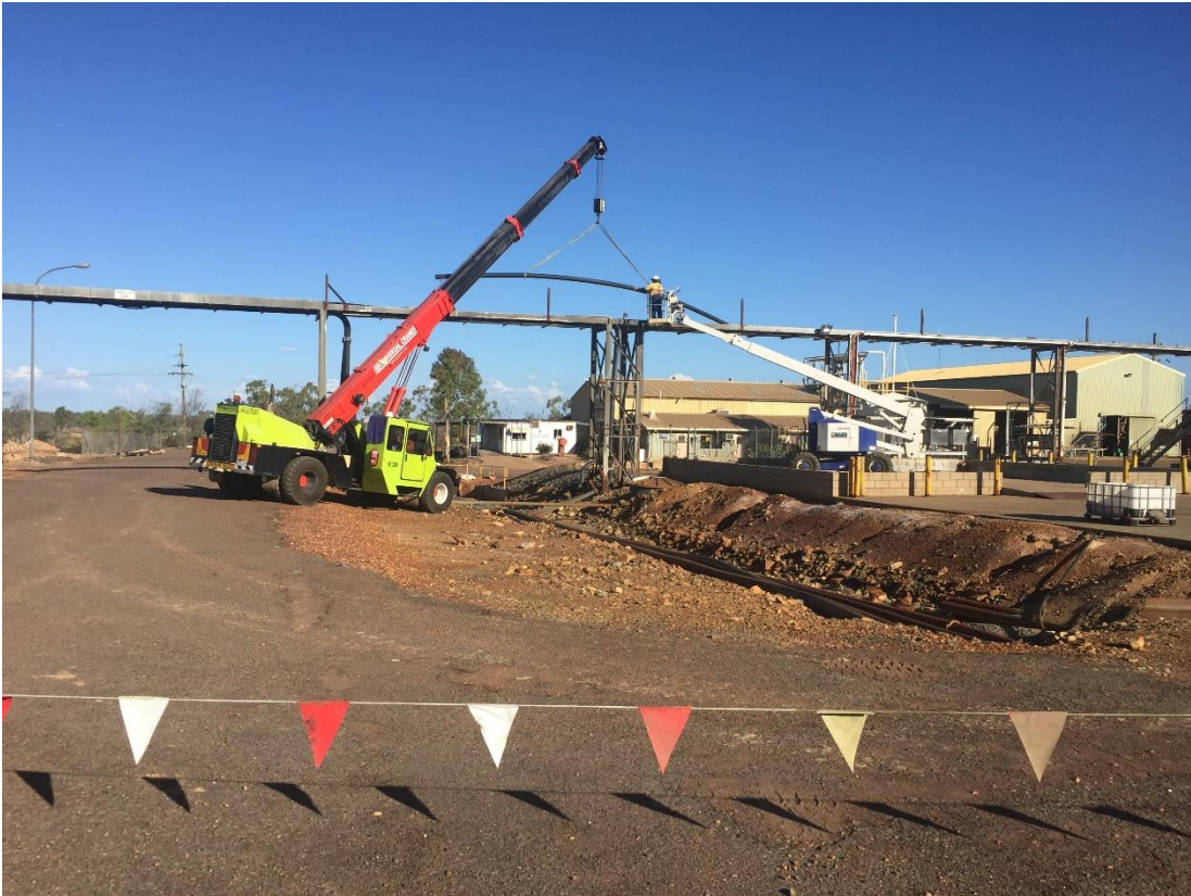
Figure 2 Overhead main raw water pipeline replacement
