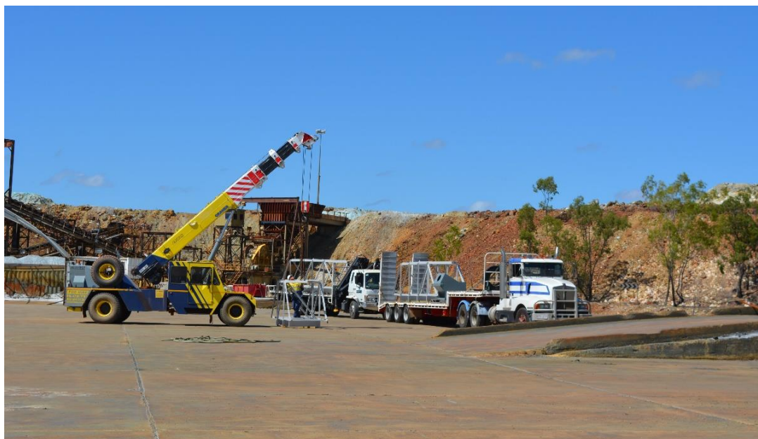
Figure 5 Unloading thickener rakes and refurbished equipment for reinstallation
