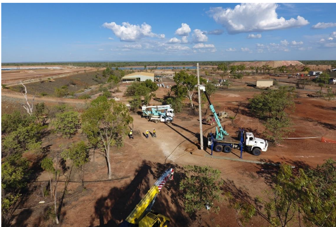
Figure 4 Replacing power poles on site
