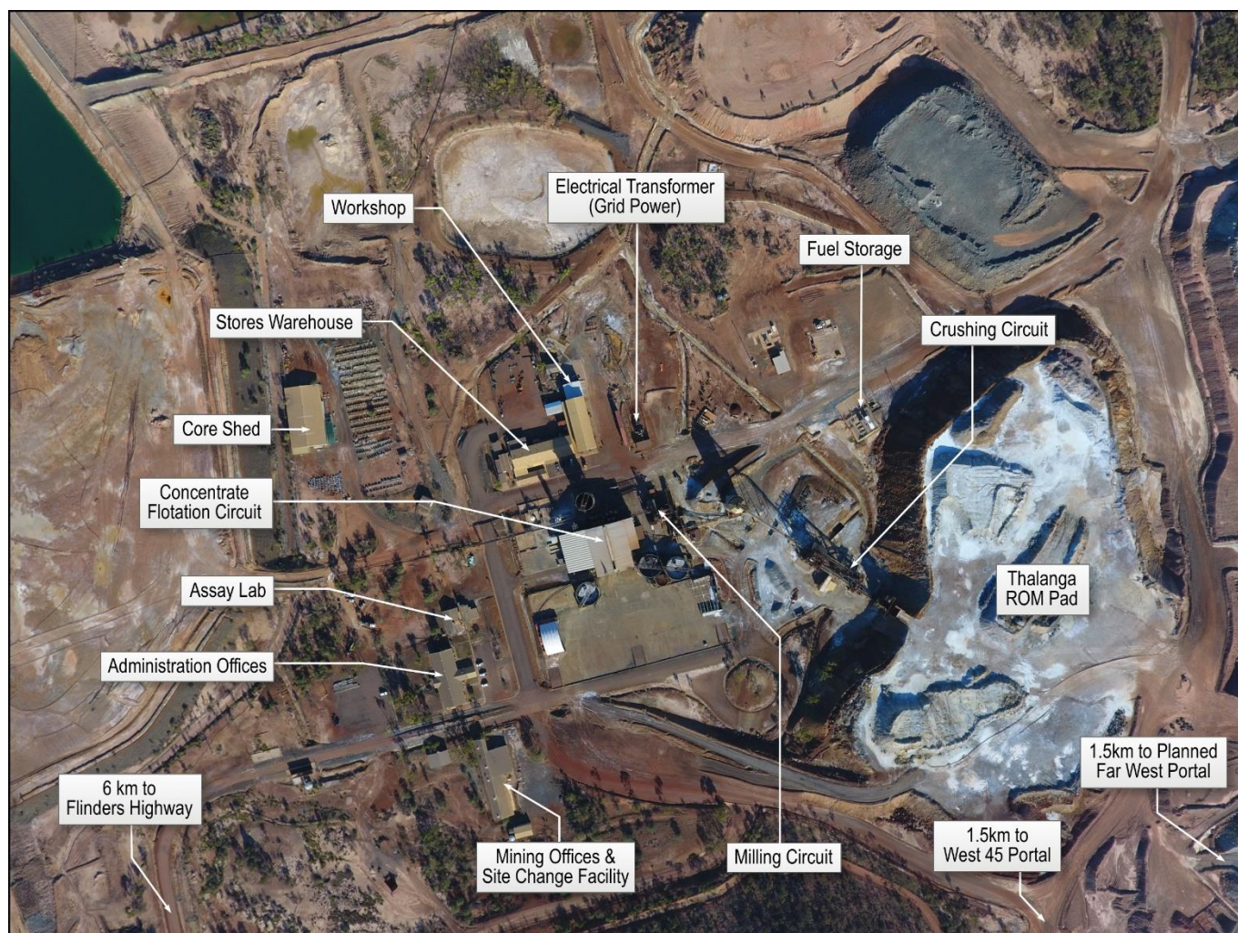
Figure 1 Thalanga Plant and Processing Infrastructure
