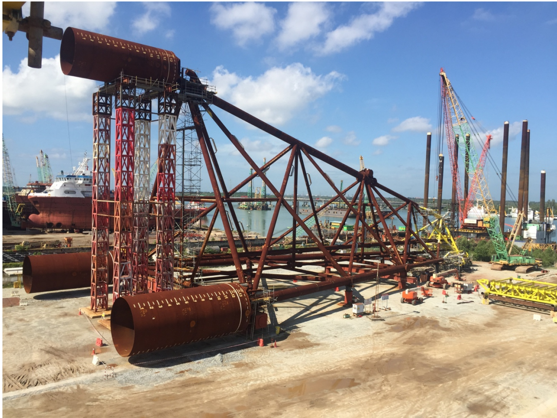
Figure 2 Ophir Jacket - showing suction piles
