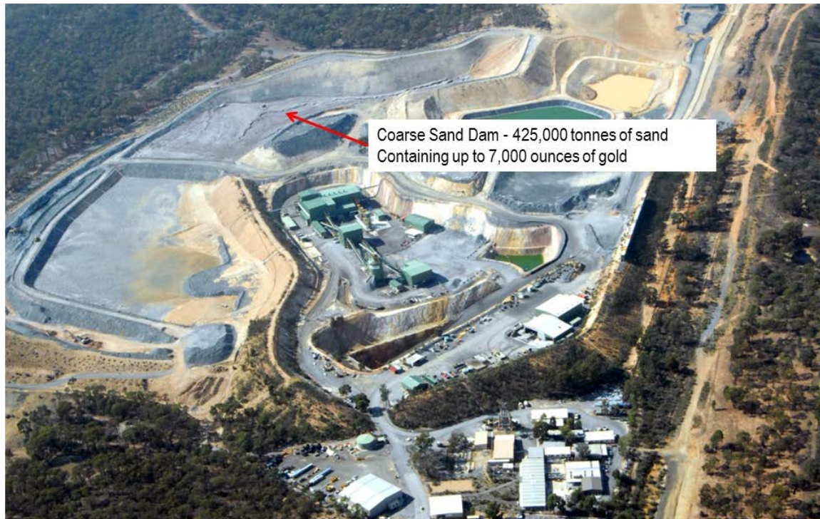
Figure 5: Coarse Sand Dam at Kangaroo Flat Mine
