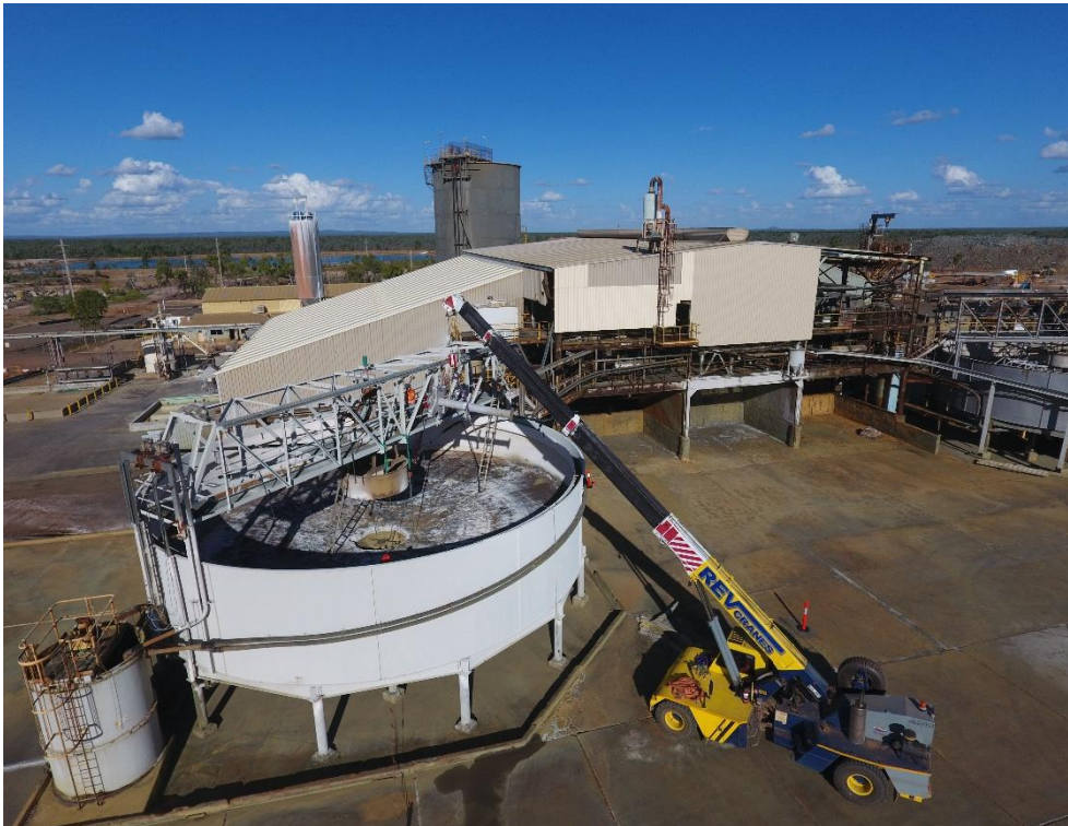
Figure 3 Replacement of shaft in main thickener
