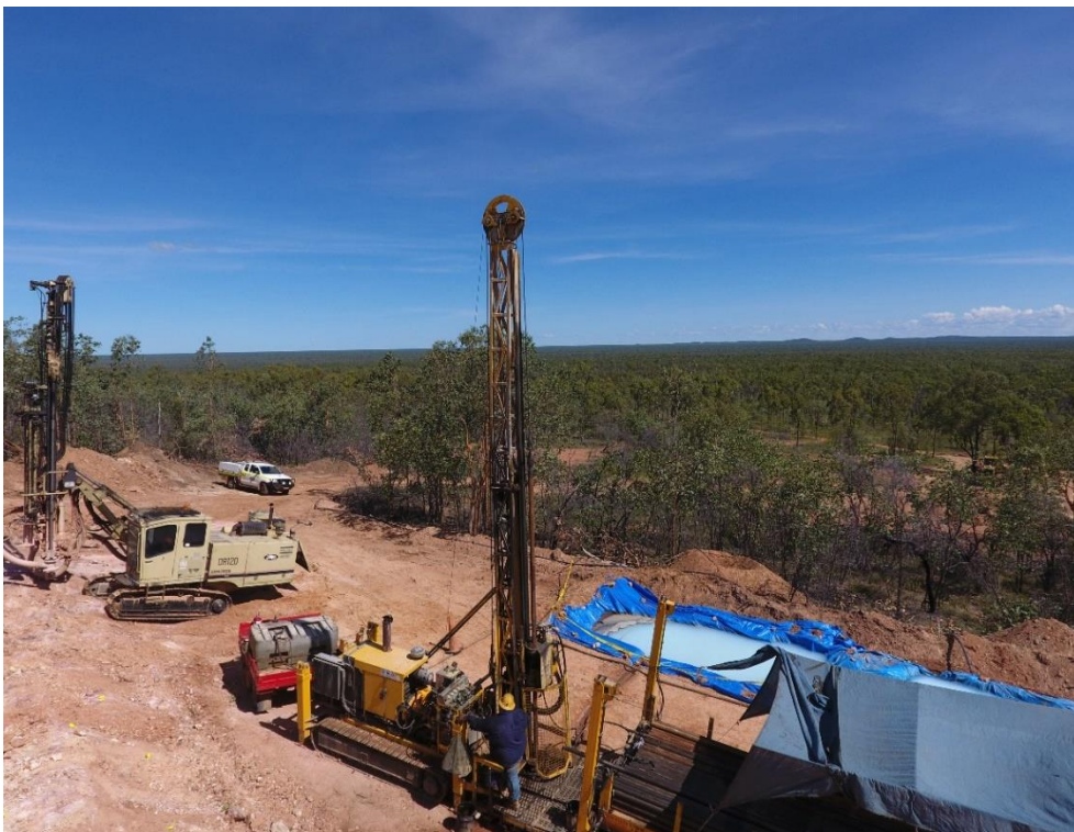
Figure 9 RAR Pad Completion Activities
