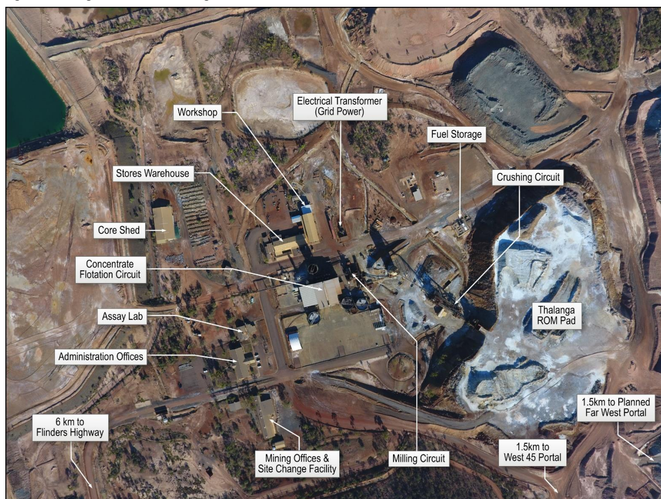
Figure 1 Thalanga Plant and Processing Infrastructure
