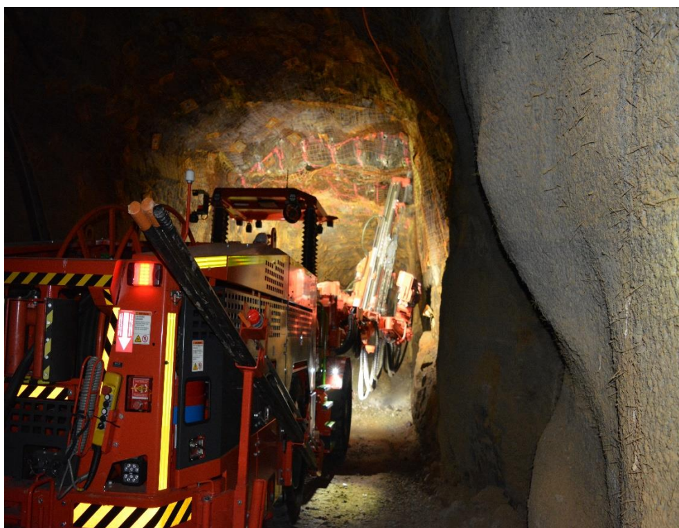
Figure 7 Rehabilitation work commenced in West 45 decline
