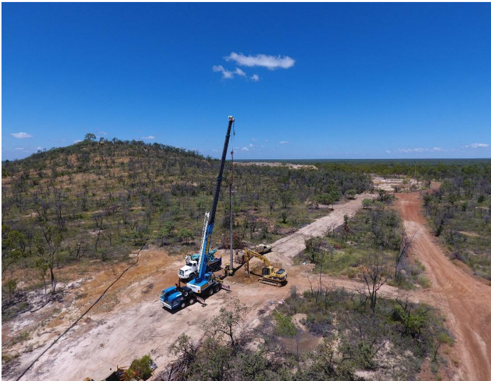
Figure 5 Installation of concrete power pole
