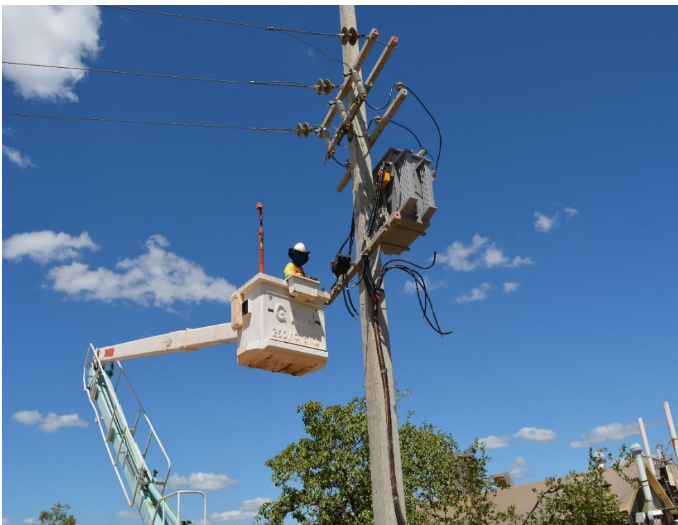
Figure 6 Installation of pole top transformer
