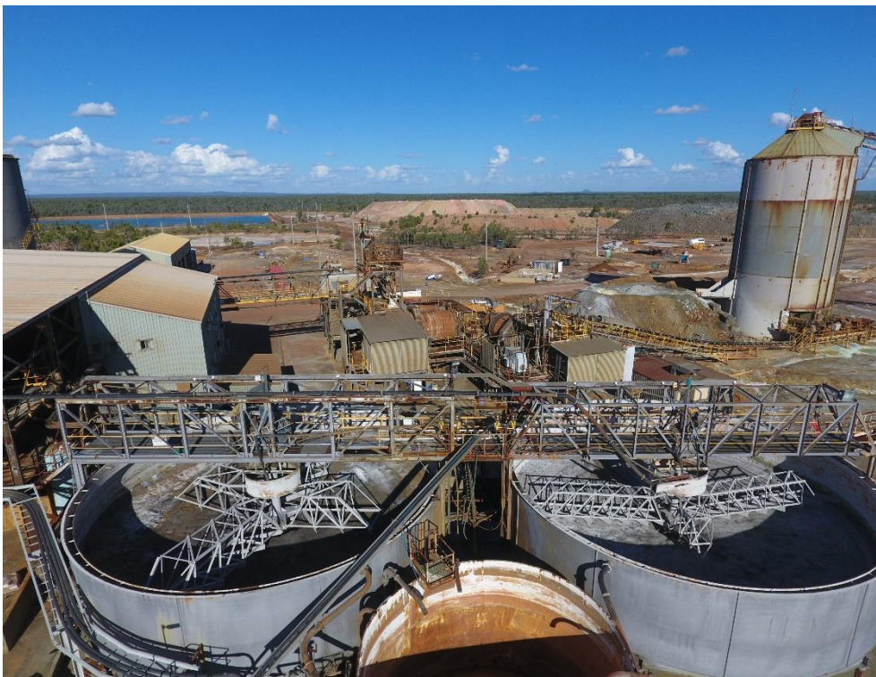
Figure 4 Installed refurbished thickener rakes
