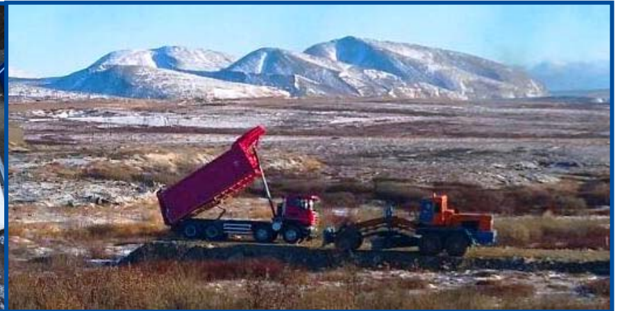
Road Construction – November 2016
