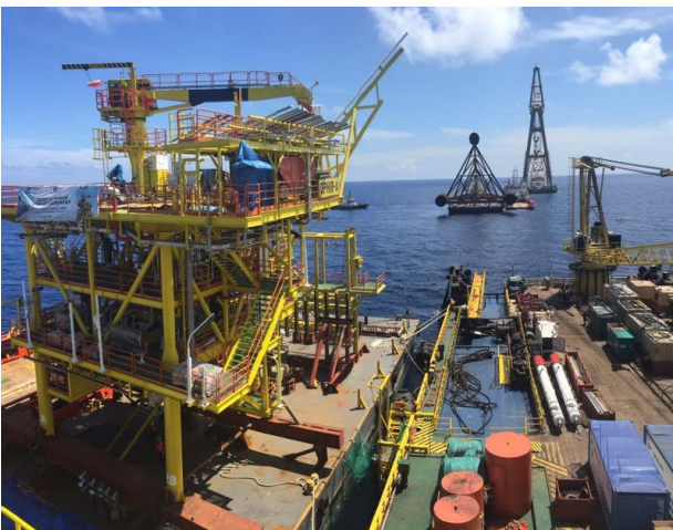
Topsides (left) aboard barge with jacket visible on barge near offshore construction barge
