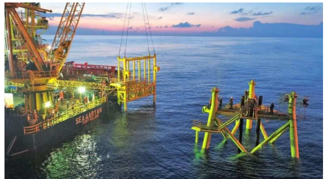
Figure 5 Ophir Platform Installation - Jacket installed, boat landing installation in process
