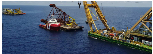
Figure 4 Ophir Platform Installation – Jacket on barge, topsides in background
