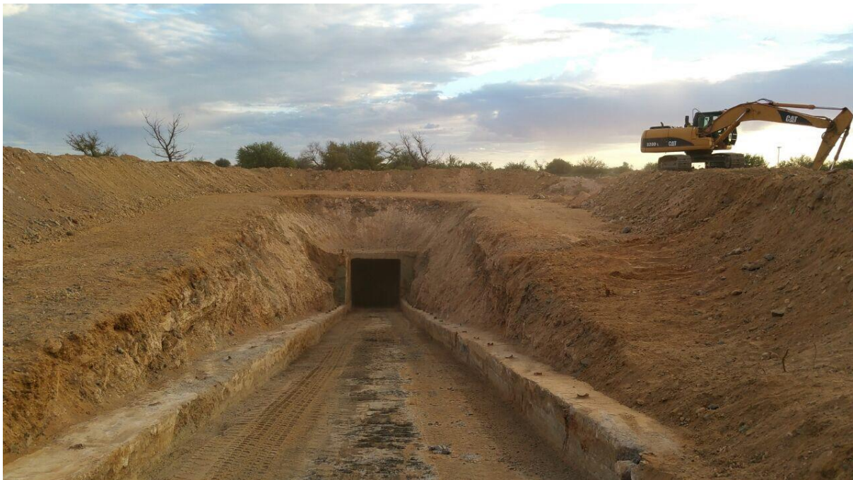
Figure 5: Refurbished decline portal at the PC Project.
