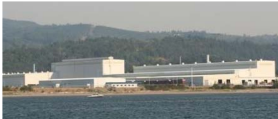
Metal coating & painting facility, Kalama, WA
