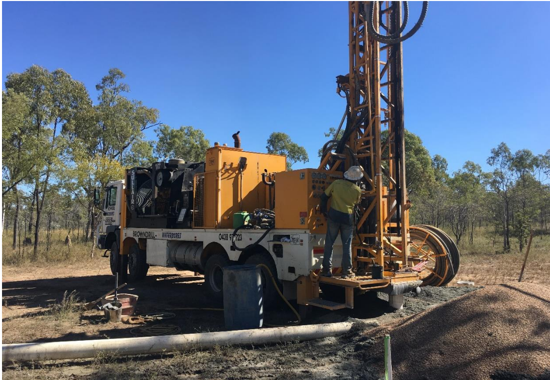
Figure 5 Installation of Far West monitoring bore
