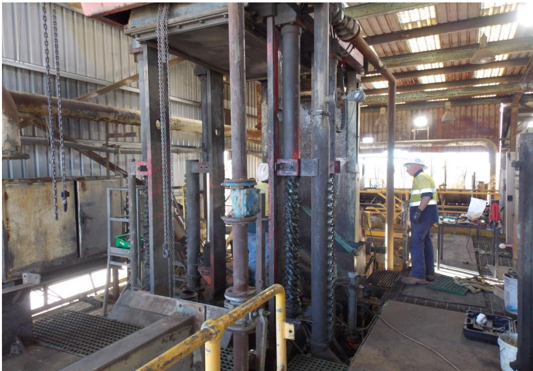
Figure 4 Ongoing refurbishment of Larox filter press
