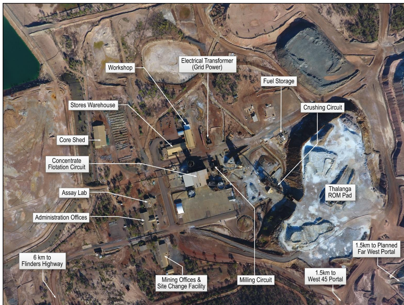
Figure 1 Thalanga Plant and Processing Infrastructure
