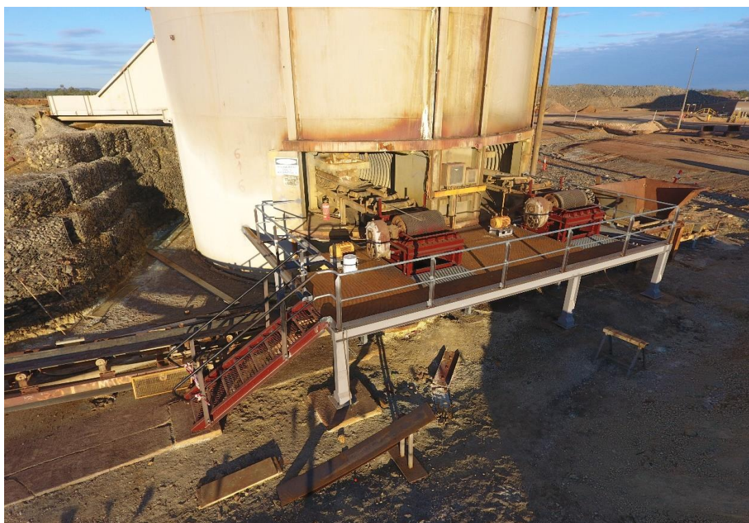
Figure 2 Replacement and refurbishment of fine ore bin feed conveyor structure
