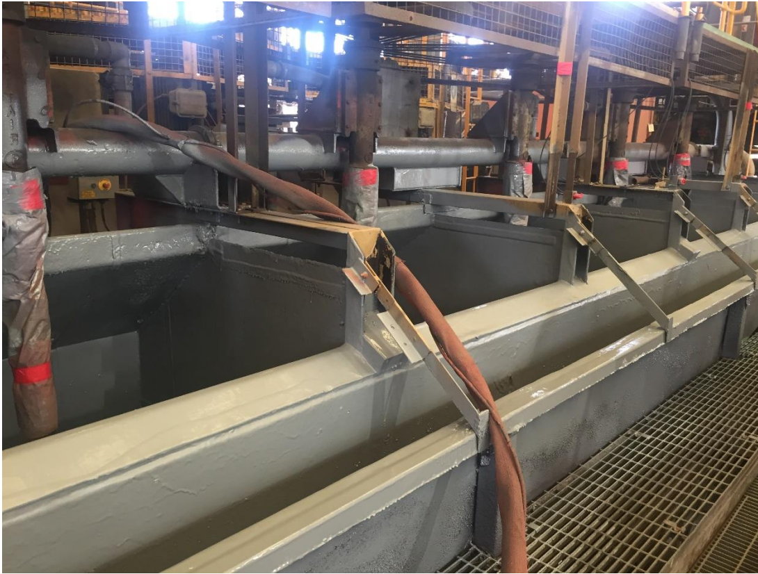
Figure 3 Repaired and poly sprayed cells in flotation area
