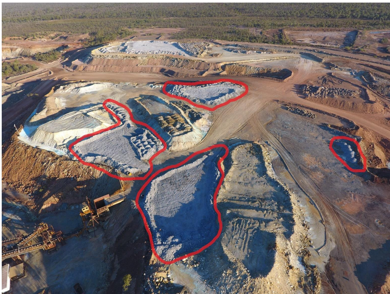
Figure 6 Thalanga ROM pad (West 45 development ore stockpiles highlighted)
