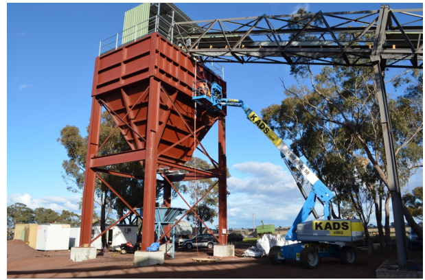
Figure 11 New outfeed hopper capable of storing 70 tonnes finished product and loading a truck in 5 minutes.
