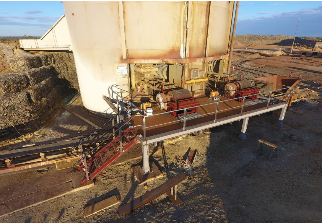
Figure 3 Replacement and refurbishment of fine ore bin feed conveyor structure
