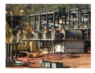
Piping, electrical connection, mechanical alignment works and grouting underway
