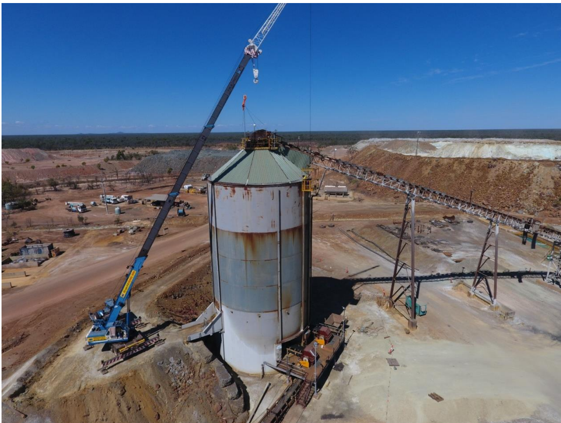
Figure 4 Fine ore bin roof installation completed
