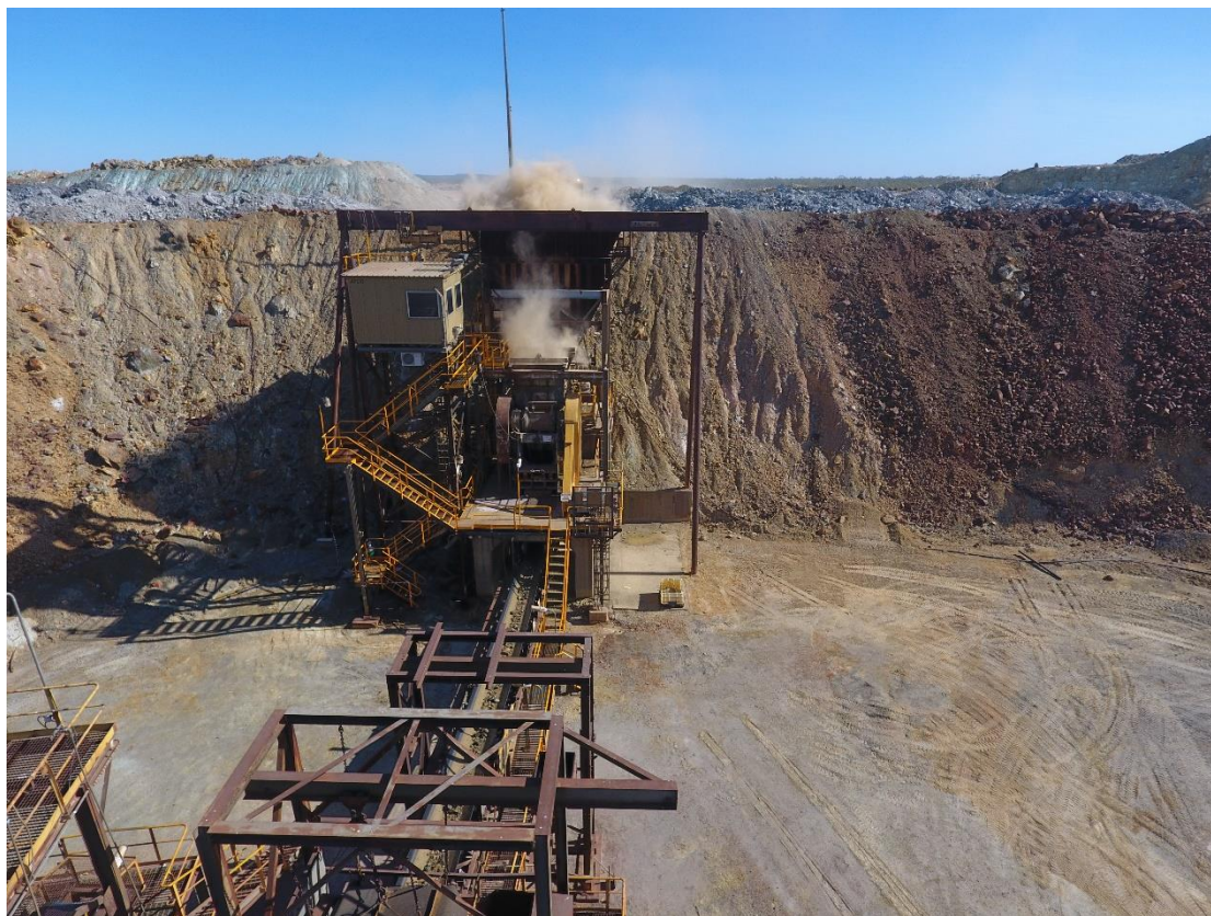
Figure 2 Crushing Circuit Commissioned and Operational
