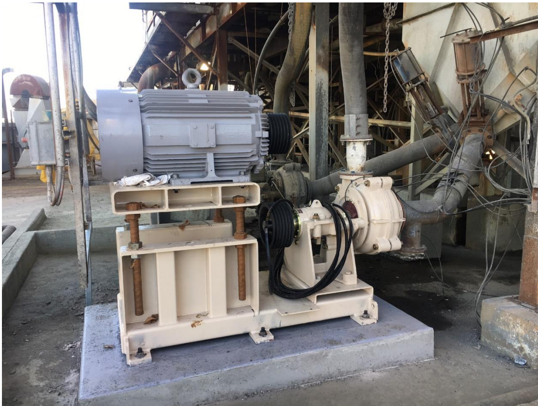
Figure 6 Tailings pump installed and commissioned
