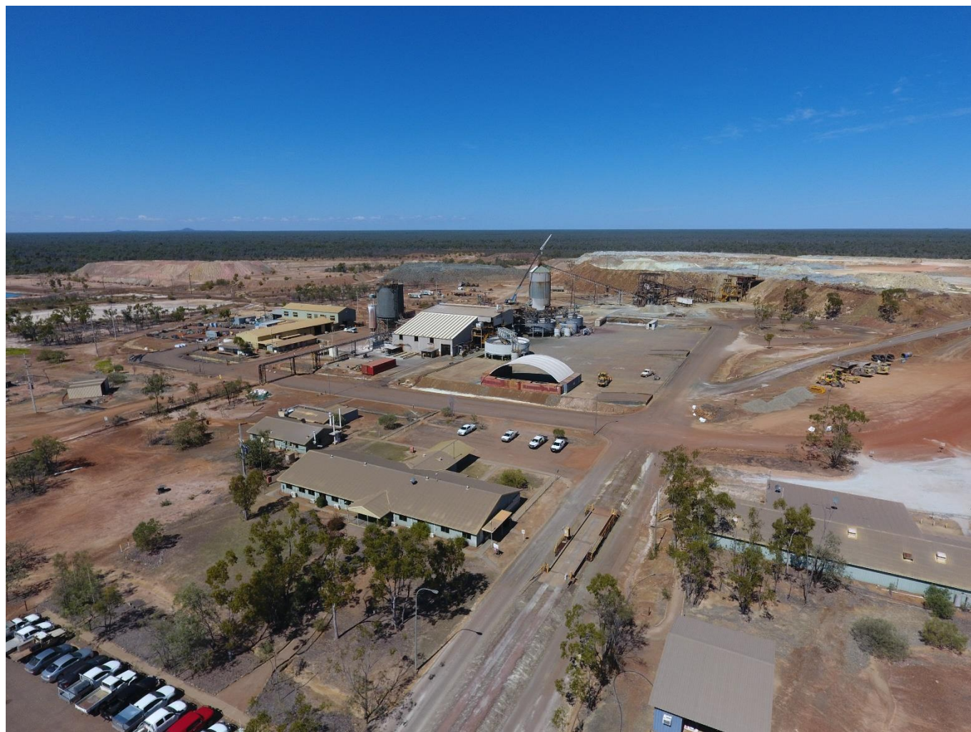
Figure 1 Thalanga Plant and Processing Infrastructure
