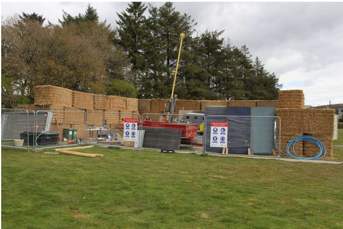
Drilling underway, with bales successfully used for acoustic mitigation
