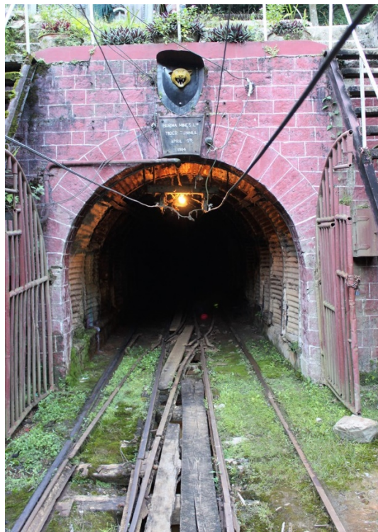
Figure 5: Tiger Tunnel Portal, near Tiger Camp, Bawdwin
