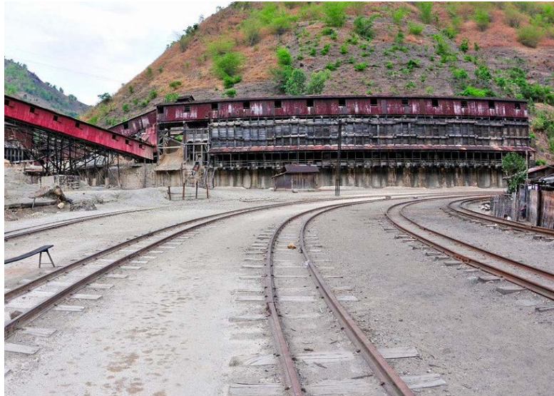
Figure 8: British-constructed ore loading facilities and rail yards provide a location for a modern grinding plant at the Tiger Camp
