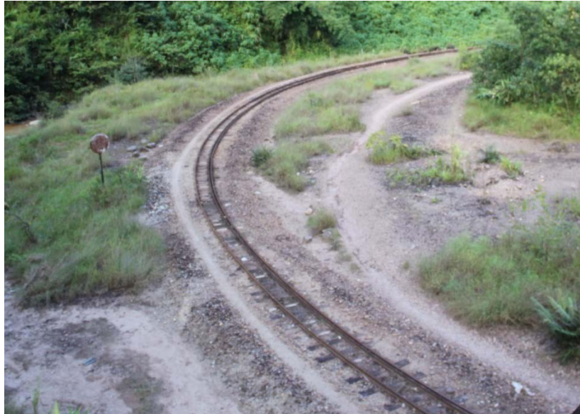
Figure 4: Narrow-gauge rail line and cleared corridor runs 15 miles from Bawdwin to Namtu
