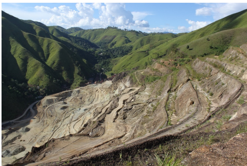
Figure 3: Bawdwin open pit looking north, ready for extension by cutting back the east wall
