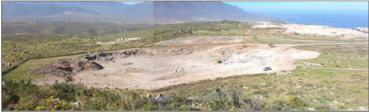
Figure 4 - Development of mine pit looking south - shows first major bench completed October 2017
