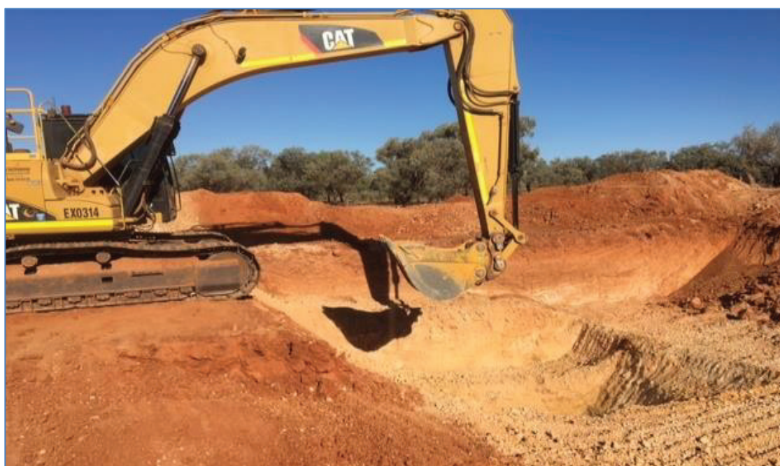
Figure 7. Excavation of 2016 Sample 2 at the site of drill hole ARC647. The pale, beige material is shallow phosphate.
