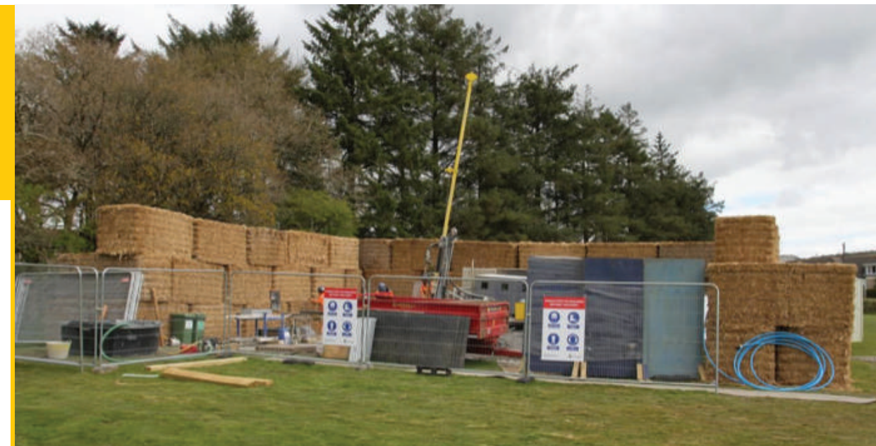
Drilling underway, with bales successfully used for acoustic mitigation
