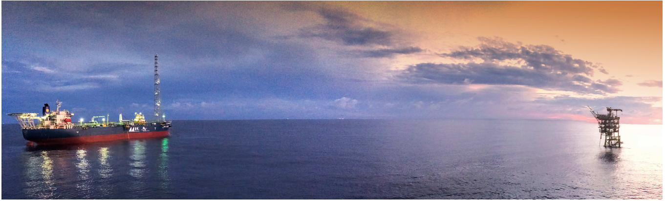
MTC Ledang FPSO and Ophir wellhead platform
