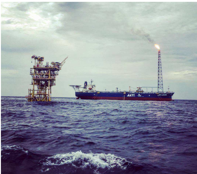
Ophir wellhead platform and MTC Ledang FPSO
