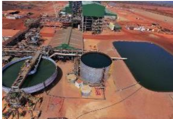
Process water storage
