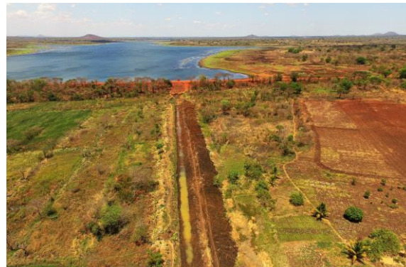
Chipembe Dam irrigation channel and agricultural land clearance and cultivation for crop planting
