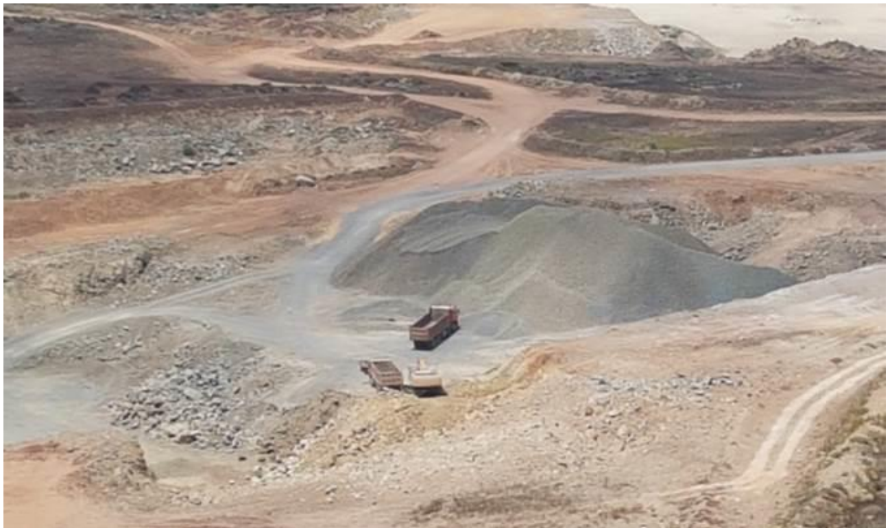
Figure 1 – In-pit crushed ore stockpile produced during the testing of a contract mobile impact crusher
