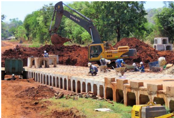
Chipembe Dam installation of concrete culvert on spillway.
