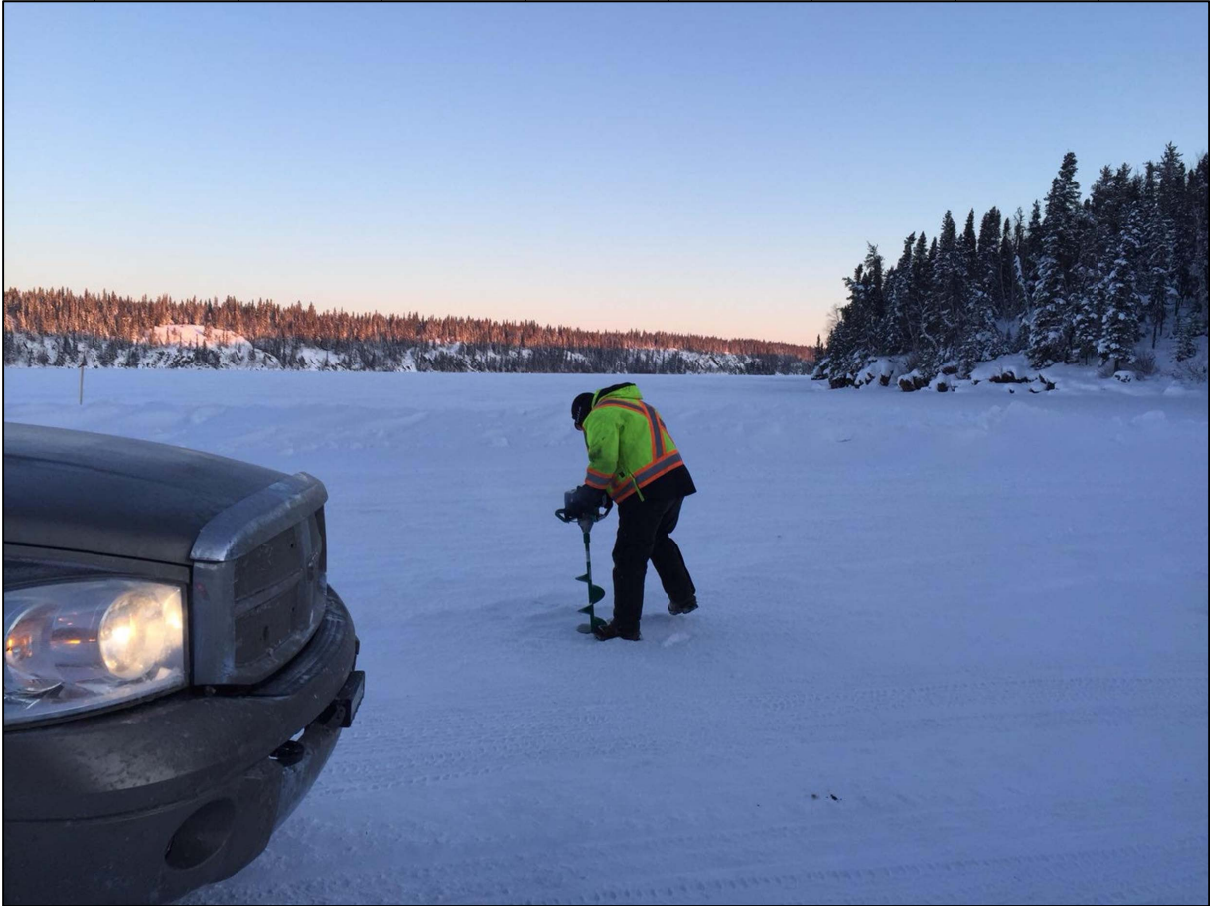
Figure 5: Thompson Bros. Lithium Project ice road access route being tested for integrity to haul drilling rig and ancillary support equipment
