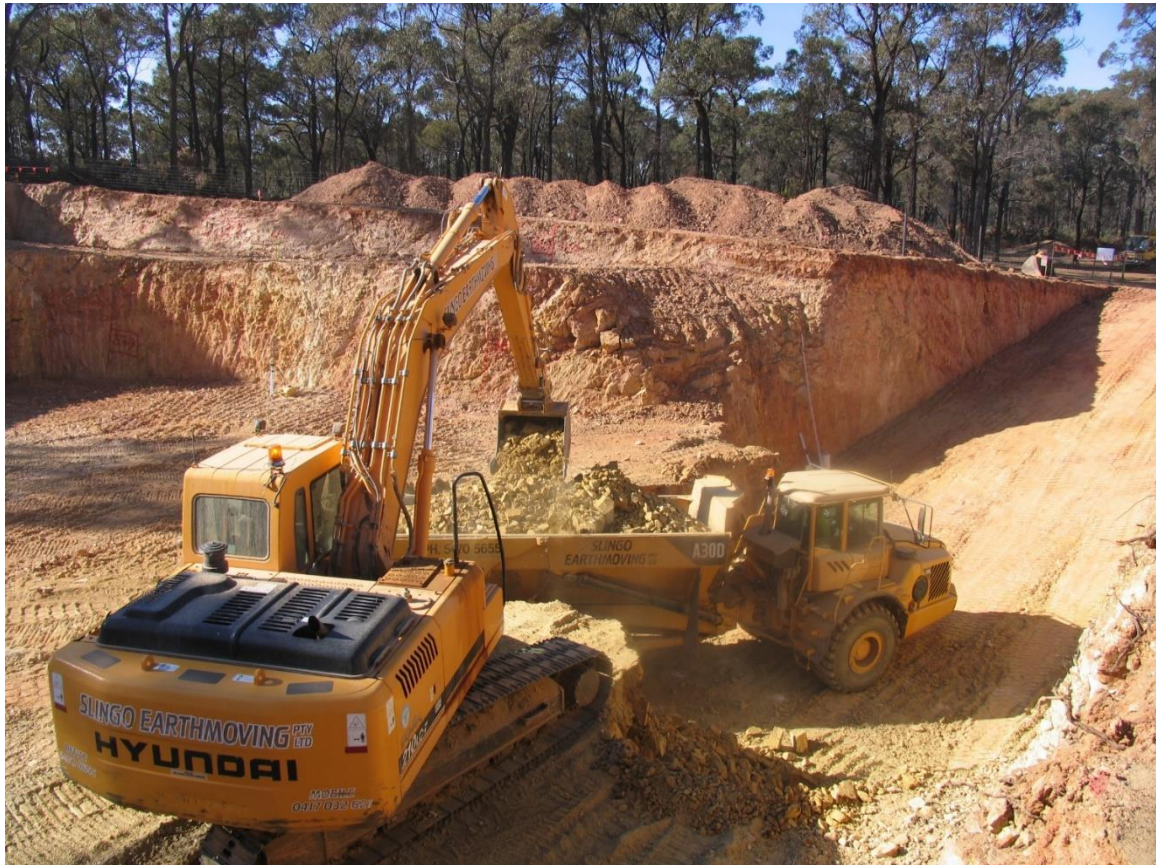
Figure 6: Excavating Bulk Sample Pit at Harvest Home
