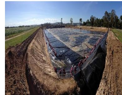
Standard prawn ponds have to be levelled and lined with protective sheeting. Yamba ponds fully operational for Novacq™ production
