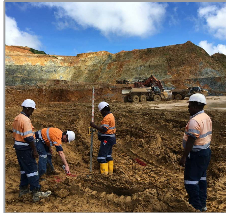
Survey work in Sorowar pit, October 2017
