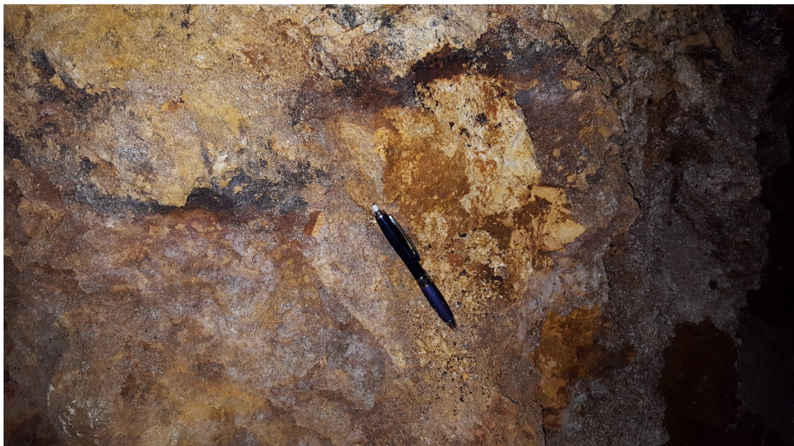
Oxidised base metal sulphides in a historical adit, Gold Hole Valley. Image: Valentis Services
