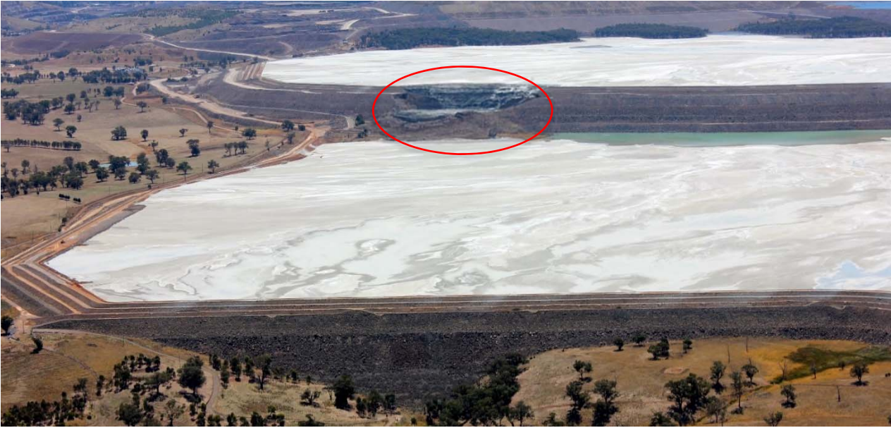
Photo of the Northern and Southern (forefront) Tailings Dams at Cadia
