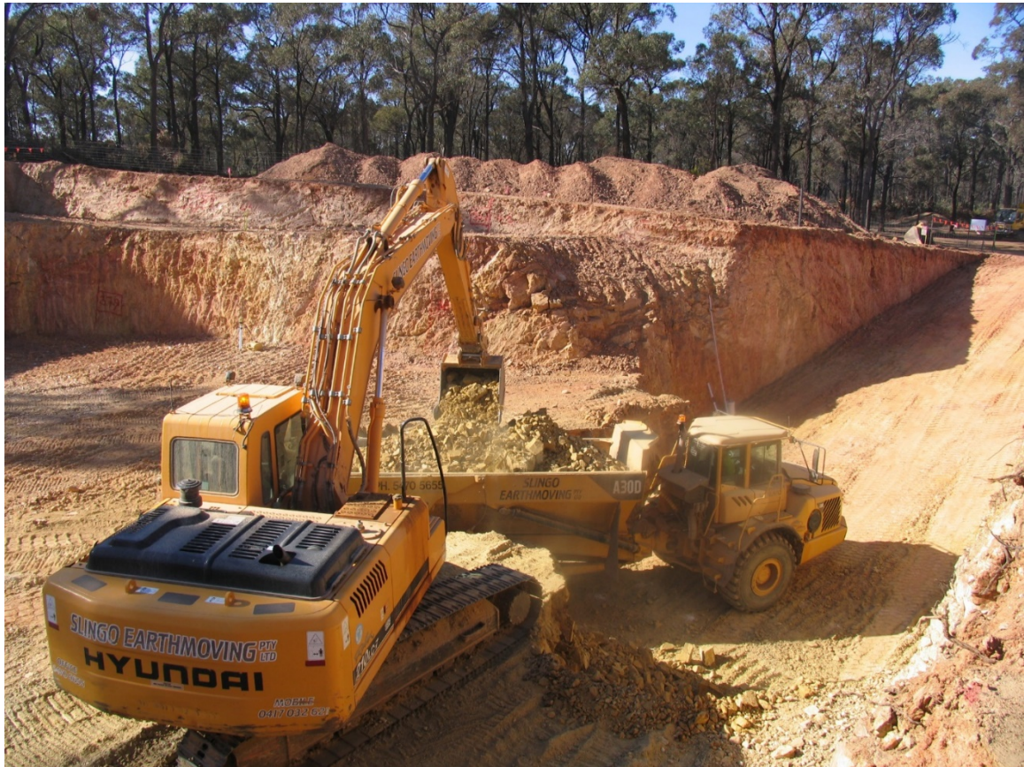
Figure 5: Excavating Bulk Sample Pit at Harvest Home
