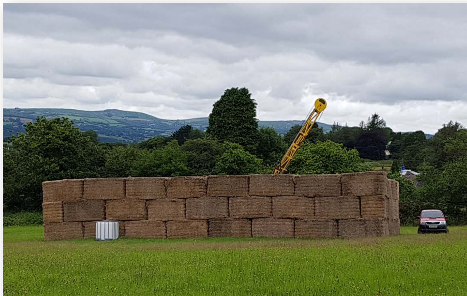
Straw bale noise screen to minimise disturbance
