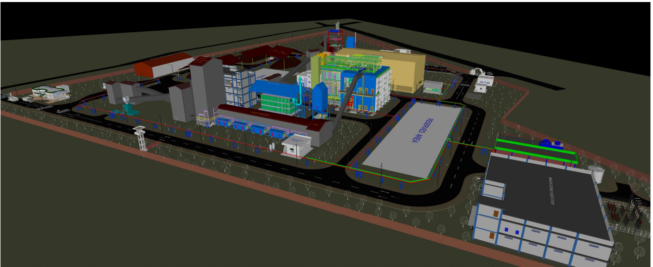
Above: a view from the northeast shows the main substation in the right-hand foreground. The reserved area allows for future expansion of the Coldry plant.
