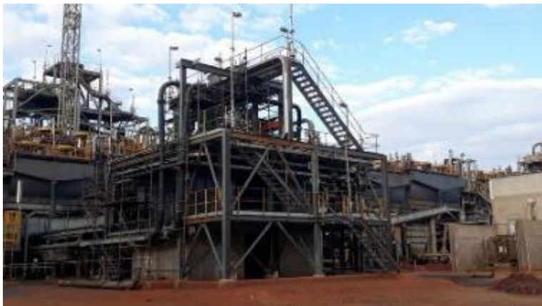
Fine flake circuit attrition cells
