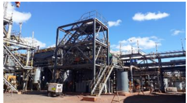
Coarse flake circuit attrition cells
