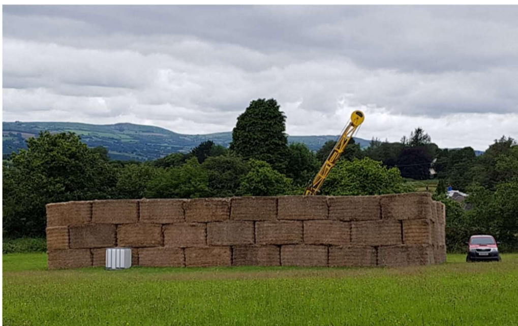
Figure 8 - Drilling underway, with bales successfully used for acoustic mitigation
