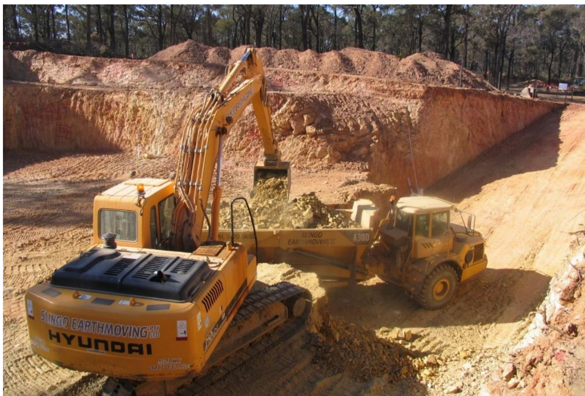
Figure 3 - Excavating bulk sample pit at Harvest Home
