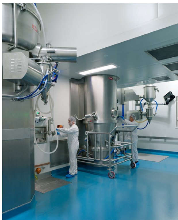
Top image: Roof space above new manufacturing extension in Salisbury Bottom image: New SMA production suite for high volume granulation and drying product process in Salisbury
