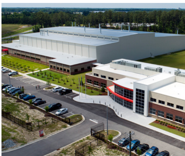
New solid oral dose manufacturing facility together with the new employee / visitor centre containing conference rooms, training space, cafeteria and fitness centre in Greenville, North Carolina
