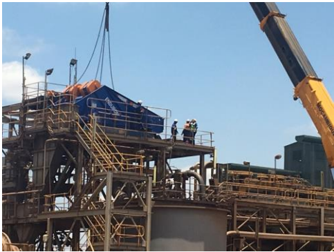
Replacement Primary Classifier Unit in place
