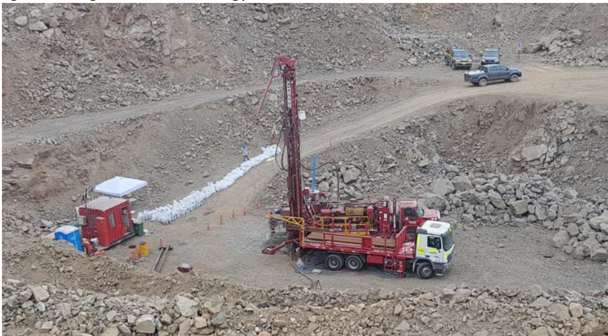
Figure 2 – Drilling inside base of trial mining pit
