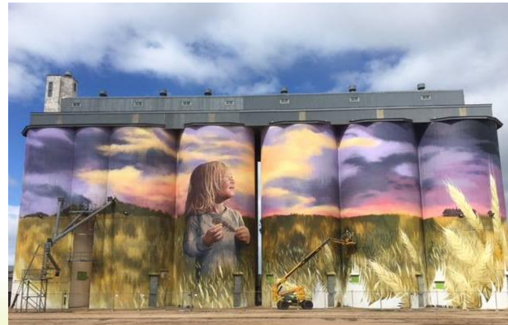
Painted Kimba silos
