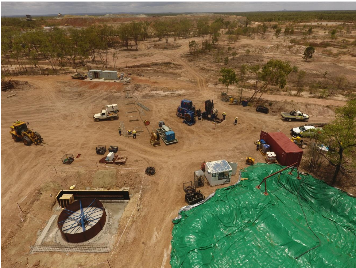
Figure 4 Far West Return Air Rise Site Preparation (Raise Borer located on Emergency Egress Pad)
