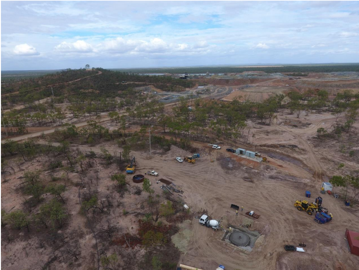
Figure 4 Far West Return Air Rise Site Preparation (Raise Borer located on Emergency Egress Pad)
