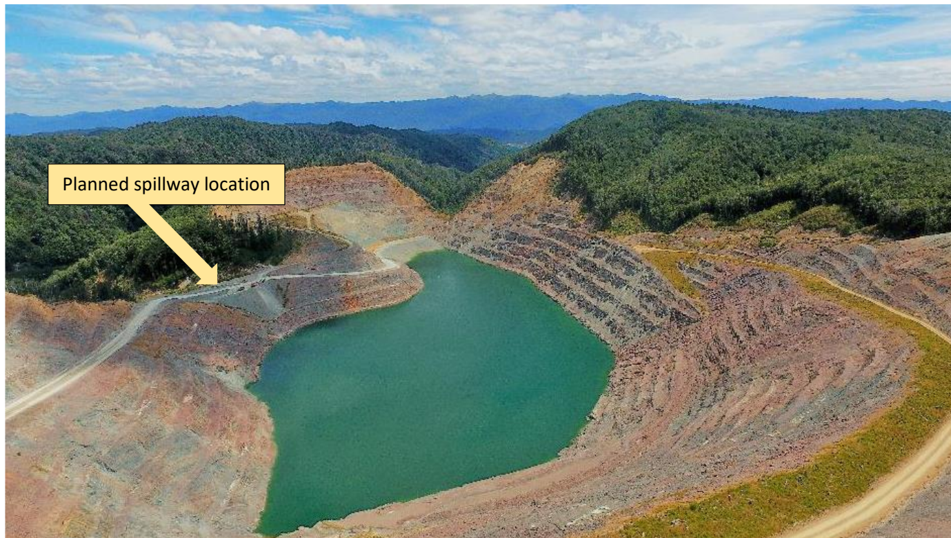
Figure 3 – Globe Pit Rehabilitation
