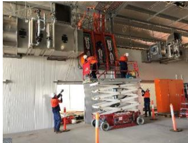
Air handling units for growing rooms
