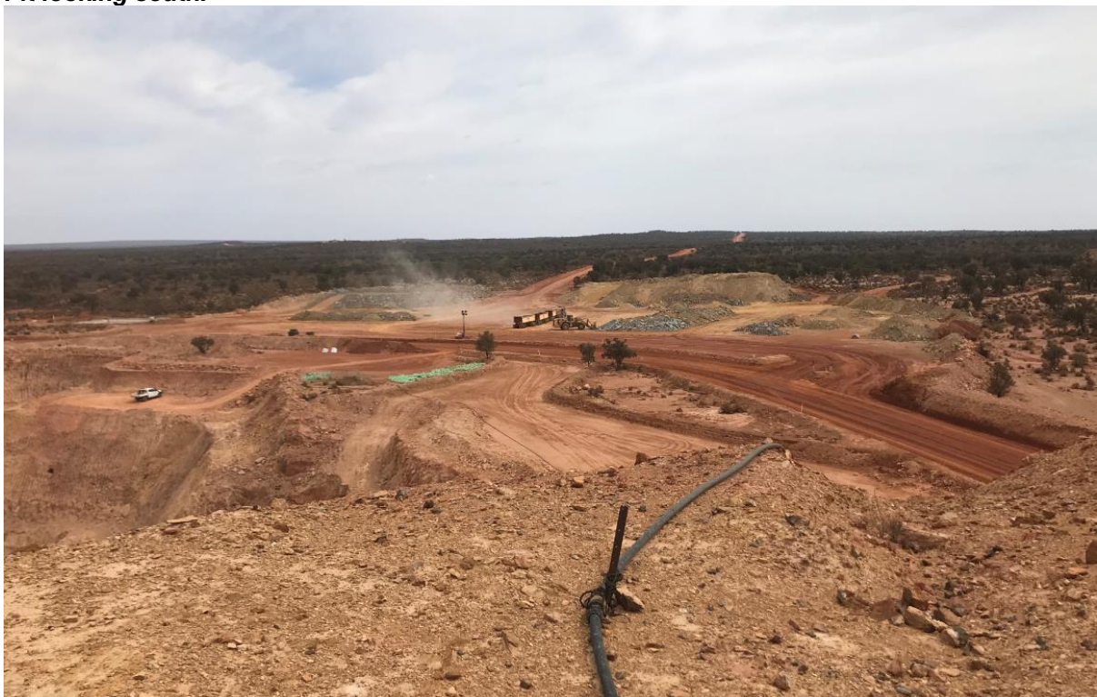
ROM Looking North.
